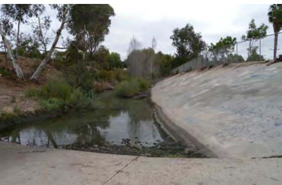
Stormwater swales and permeable paving (top and middle) allow water to infiltrate, preventing polluted runoff from entering streams (bottom).
